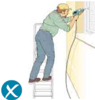
Figure 7a Incorrect - steps side-on to work activity
